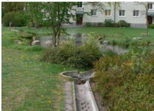
Fig. 7.26 swale and retention pond, Malmö, Sweden
